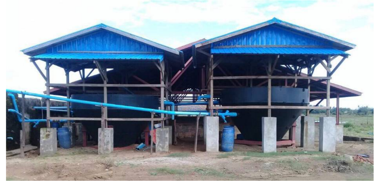
Figure 17: Hopper Bottom Tanks
