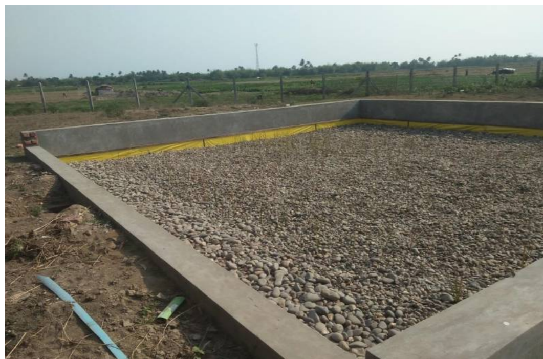
Figure 26: Secondary Constructed Wetland
