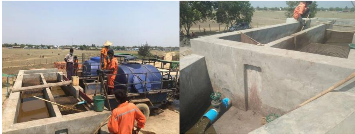
Figure 16: Emptying of tractors in the Dumping Station & Emptying of the reception tanks
