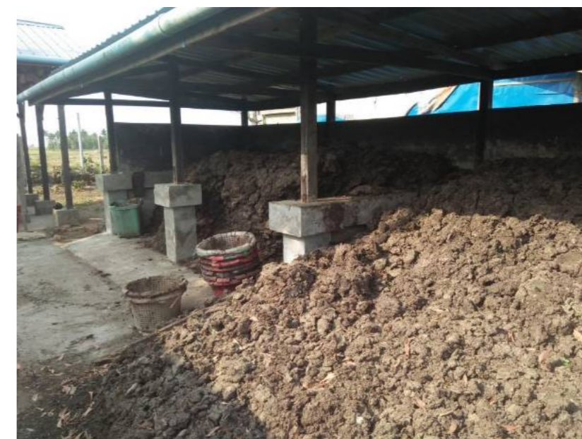
Figure 27: Dried Sludge Storage Units
