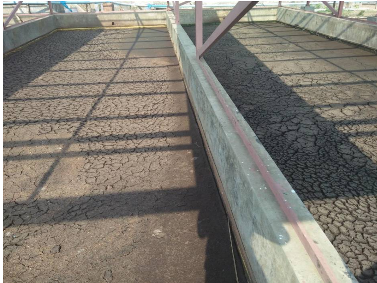
Figure 24: Unplanted Drying Beds
