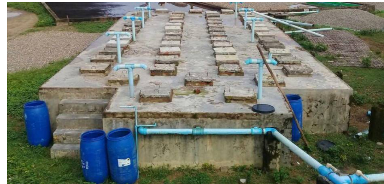
Figure 19: Anaerobic Baffled Reactor
