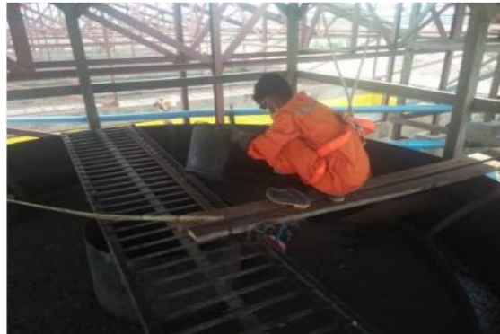
Figure 18: Scum Removal in HBT
